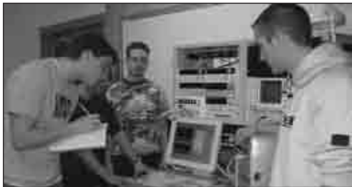
Students measuring temperature and power for competitive assessment of thermoelectric coolers.
